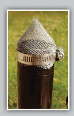
This vent pipe was screened using a fine mesh (1/16th of an inch) and secured in place with a hose clamp.
