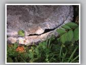
This is an example of a septic lid that is not sealed properly. Mosquitoes can easily enter through the gap.
