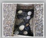
In this example the plastic does not cover the entire top of the septic. Additional sand should be used to cover the tarp as well.
