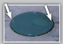
Missing screws on lid may cause a gap in the fit which could allow mosquitoes access to the septic tank.
