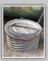
This is an example of a makeshift lid. The plywood has become warped and doesn't allow for a proper seal. The lid should be replaced with the recommended cover for this style septic tank.
