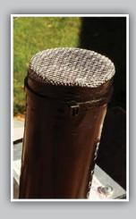
This vent pipe was screened using a fine mesh (1/16th of an inch) and secured in place using electrical tape and zip-ties.
